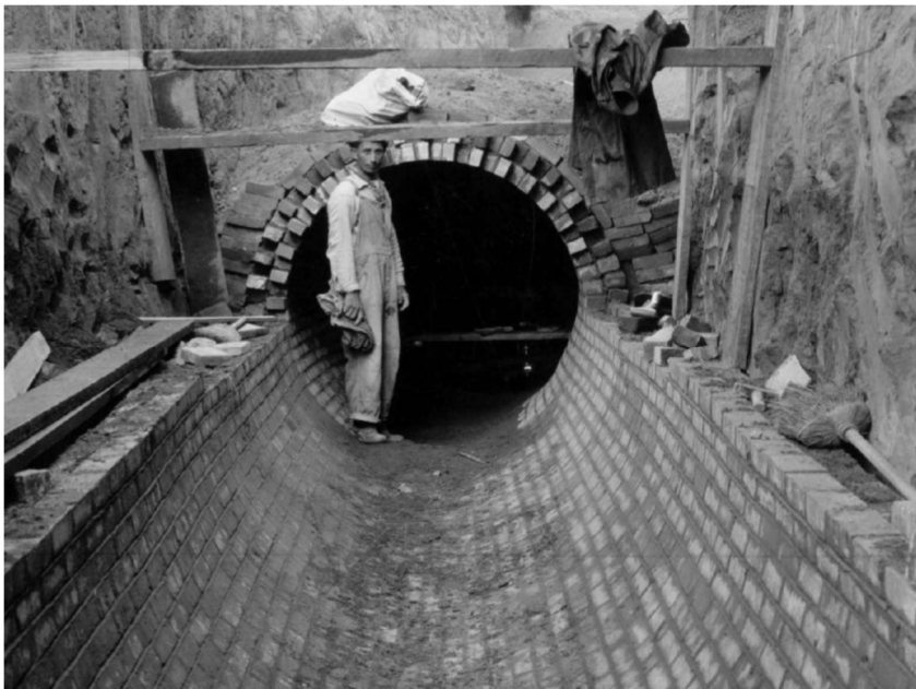
Figure 1: Construction of a brick storm drain system used to replace surface conveyance in a natural swale in the City and County of Denver circa 1920 (Denver Public Library).
