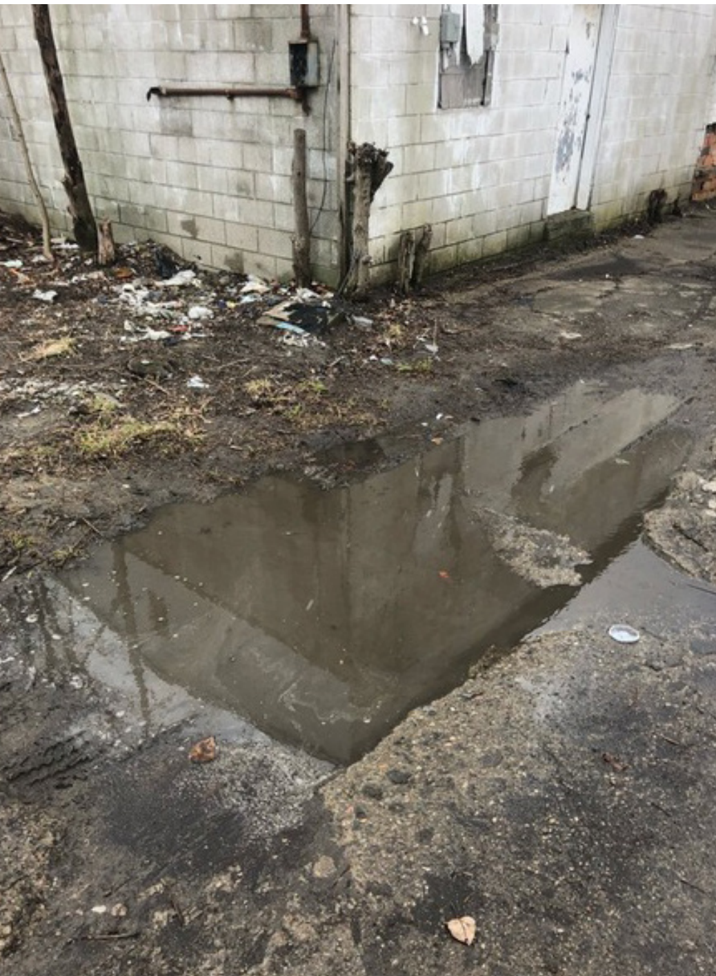
FIGURE 22. A BLOCKED CATCH BASIN IN DETROIT, AS REPORTED BY A HOMEOWNER. SOURCE: EN.SEECLICKFIX.COM.
