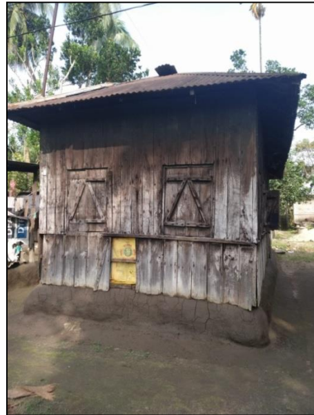
Figure 2: Raised plinth of kachcha houses
