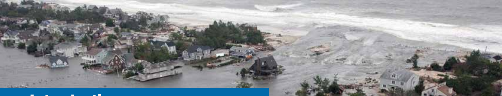
(Credit: aerial views of the damage caused by Hurricane Sandy in Mantoloking, New Jersey, New Jersey Army National Guard, Oct. 30, 2012.)
