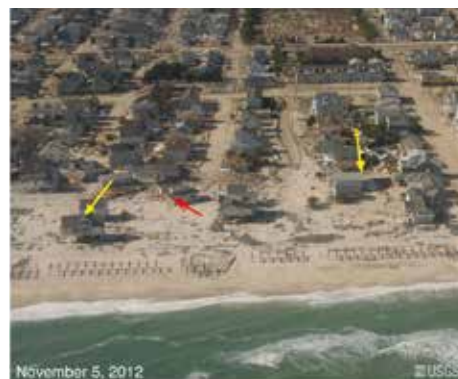
VIEW LOOKING WEST ALONG THE NEW JERSEY SHORE: Storm waves and surge cut across the barrier island at Mantoloking, New Jersey, eroding a wide beach, destroying houses and roads, and depositing sand onto the island and into the back-bay. The arrows in each image point to the same features. (Credit: images courtesy of United States Geological Survey.) 25
